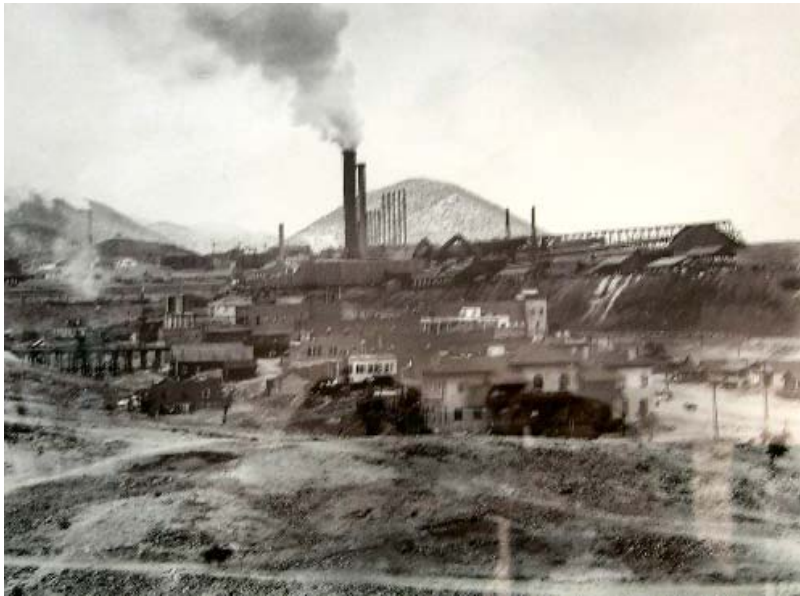
Instalaciones industriales de la Cananea Consolidated Cooper Company, 1906
